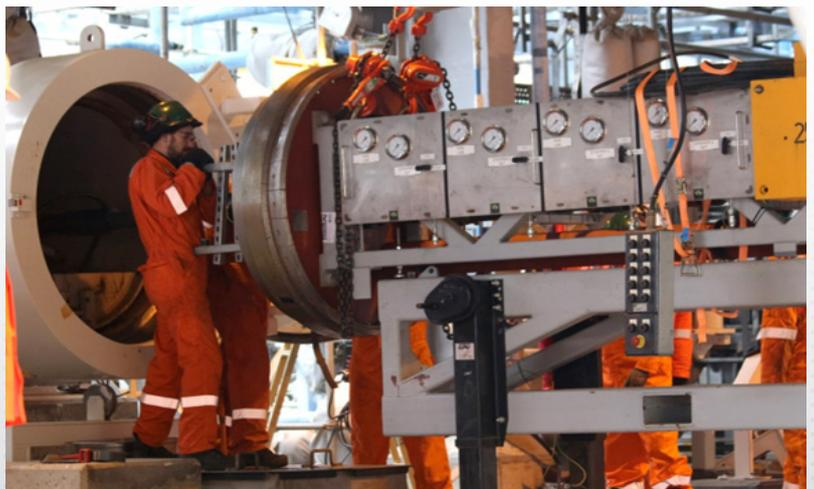
Temporary launcher door and stuffing box arrangement removal
