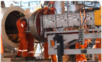
Temporary launcer door and stuffing box arrangement removal
