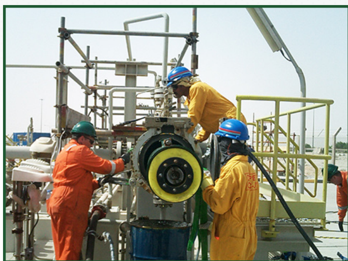
14" Remote Tecno Plug™ deployed at Natural Gas Liquids Plant (NGL-4), Mesaieed Industrial City, Qatar
