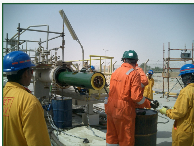
14" Remote Tecno Plug™ deployed at Natural Gas Liquids Plant (NGL-4), Mesaieed Industrial City, Qatar
