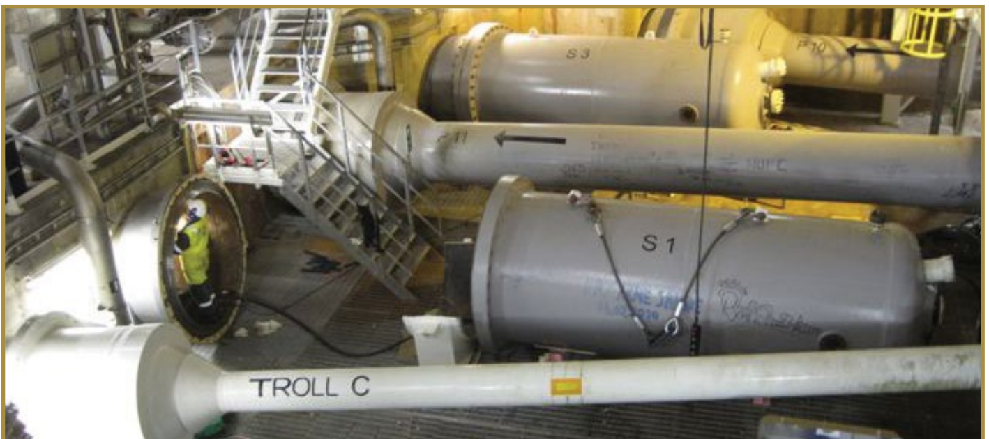
Internal End Cap removed for installation of Seal Cartridge and Temporary Anchor
