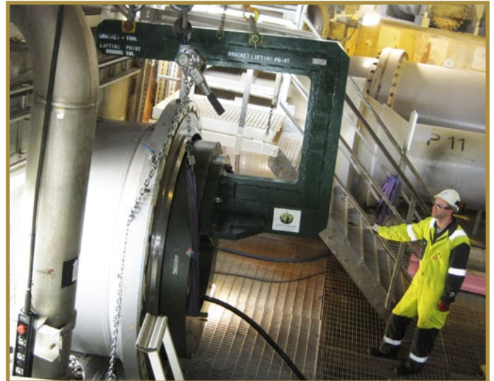
Seal Cartridge installation
