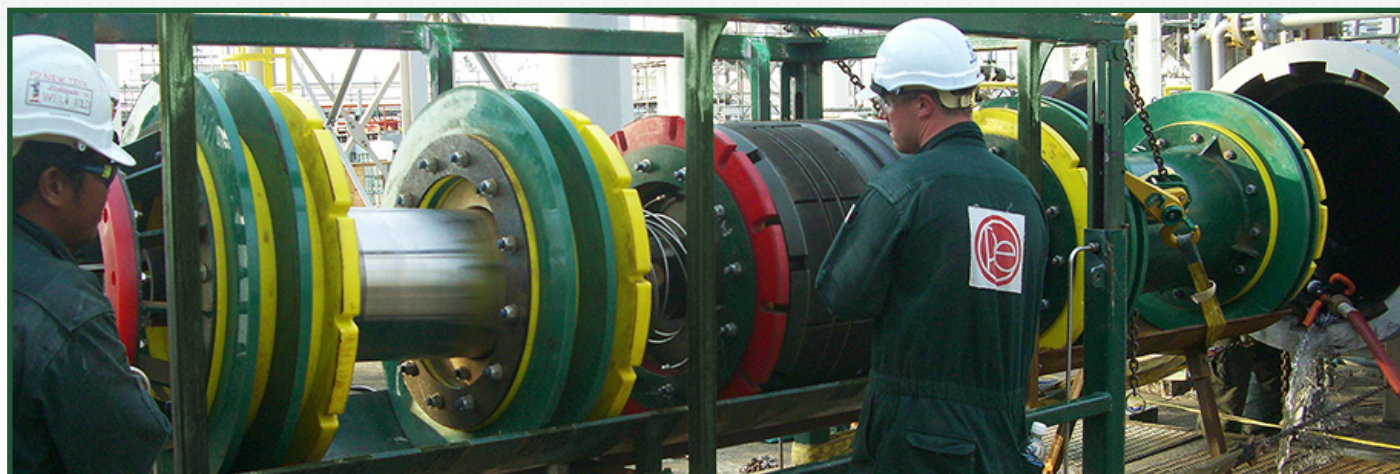
STATS isolation technician Iain Reid, prepares 36" Remote Tecno Plug™ for deployment
